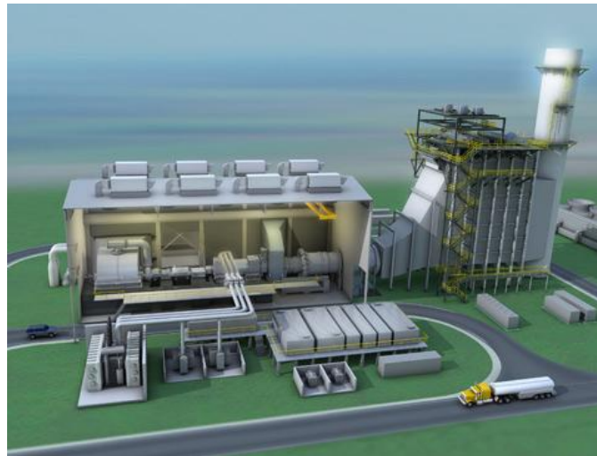
Figure 3. Combined cycle gas turbine power plant
