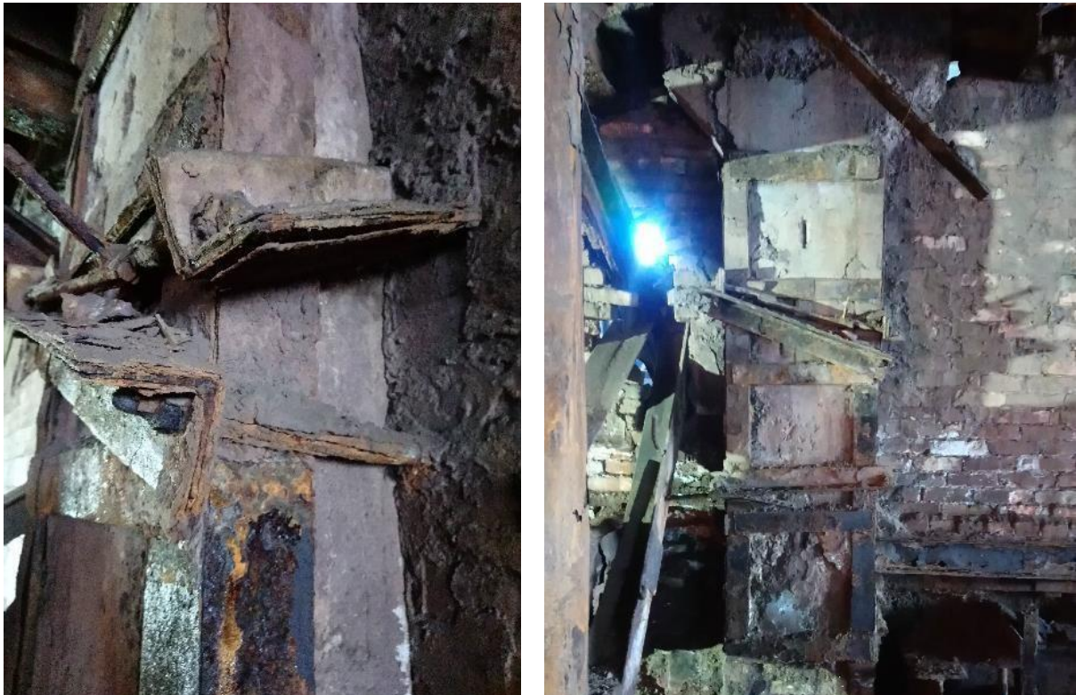
Figure 3. Column along the axis of 6-B
